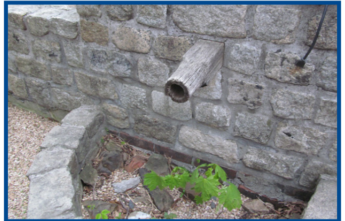
In the photo, an old abandoned water main dates to the Civil War era.
