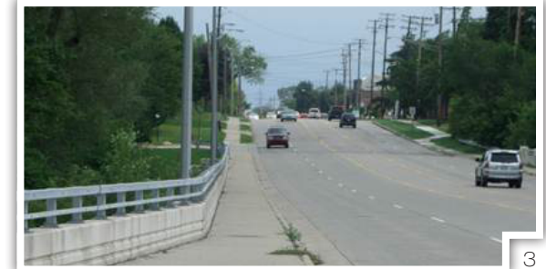
Bridge Over Rouge River
