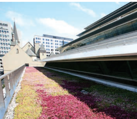
Grand Rapids' UGI requirements are playing a key role in site design. Green roofs, in particular, are more widely utilized as a method of meeting the greenspace requirement in commercial districts.
