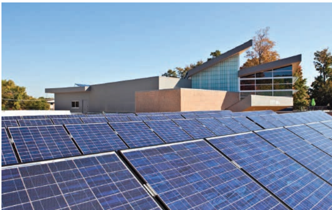
Energy costs at city hall have been slashed through the use of photovoltaic panels, a solar hot water heater, and a ground source heat pump system. The city realized a 54 percent reduction in utility-derived energy and a reduction in energy costs of 37 percent.
