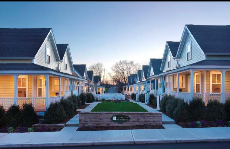
Inward views to stormwater-catching court
