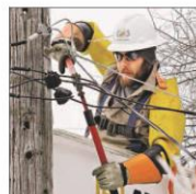
Cory Bean repairs a line Thursday in East Lansing. AL GOLDIS/AP
